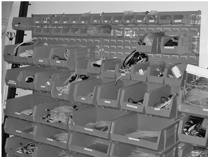
Figure 6.16 Various sizes of labeled blue bins are used to store a variety of data center supplies at GNAC, Inc.
