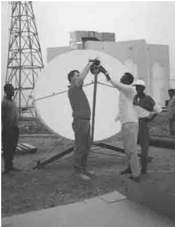
Figure 2-12 Workers set up a fly-away satellite uplink. (Courtesy of Earth Stations)
