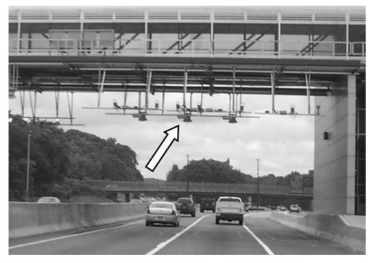
Figure 1.10 E-ZPass High-speed Toll Plaza–Antenna Array
